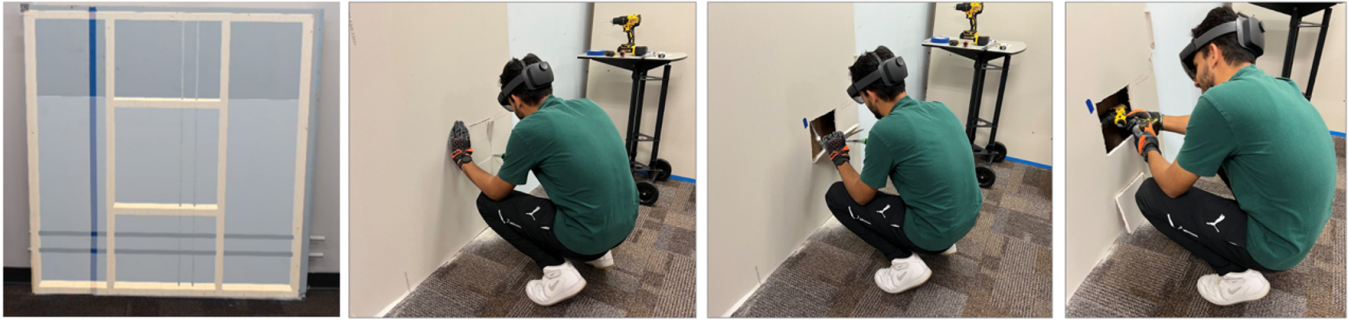
Figure 2: Using an AR+BIM L1 headset to guide an electrical outlet wiring and installation task. (1) The testing apparatus for the experiment overlaid with the augmented view behind the wall, (2) the participant aligns the AR-guided placement on the wall; (3) AR guidance supports cutting the drywall opening for the outlet box; and (4) the participant installs the electrical box following the AR instructions. The AR system provides both spatial guidance and L1 instructions to assist with accurate placement and step-by-step completion of the installation procedure.
